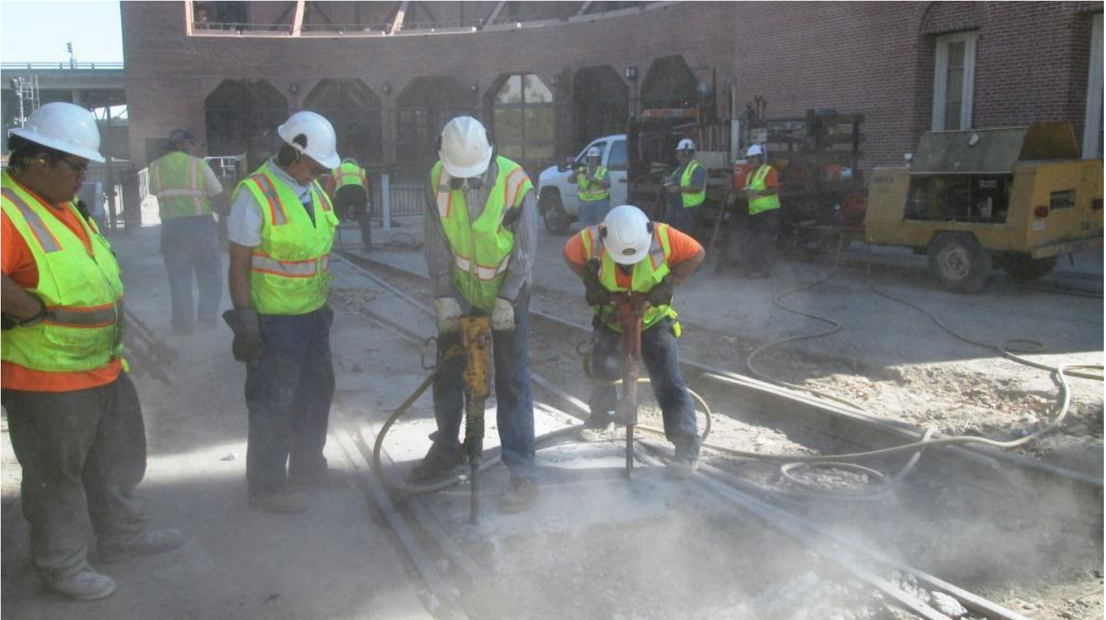
Steve and Joe are the next to experience some quality time with the jackhammers
