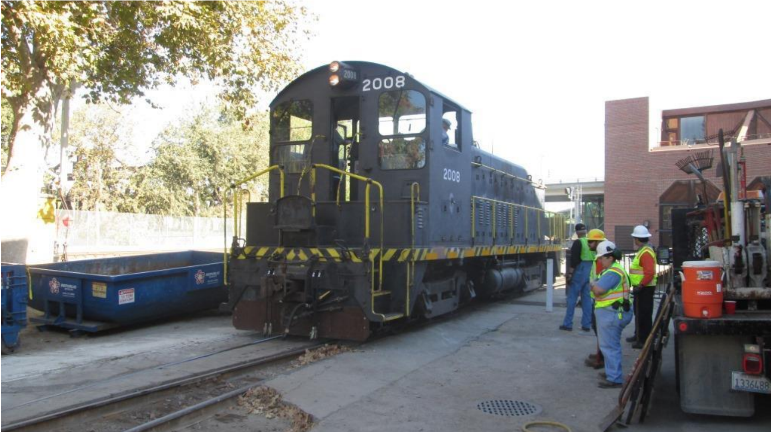
Once the locomotive is out of the way, the Team can really go to town on tearing up concrete
