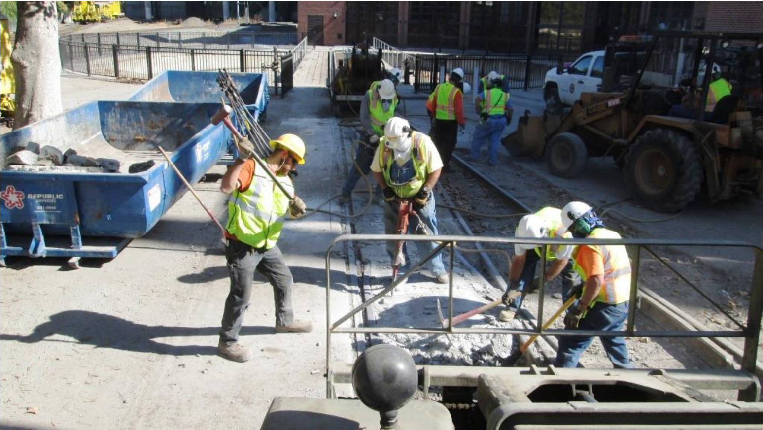
Chris M. employs a sledgehammer and Clem and Joe use mattocks to break up the concrete within the frog. Mike F. and Steve use jackhammers and work into the frog from the north
