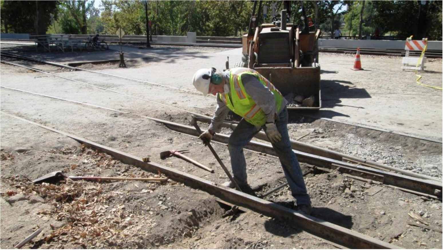
Steve tightens down a clamp on a gauge-rod
