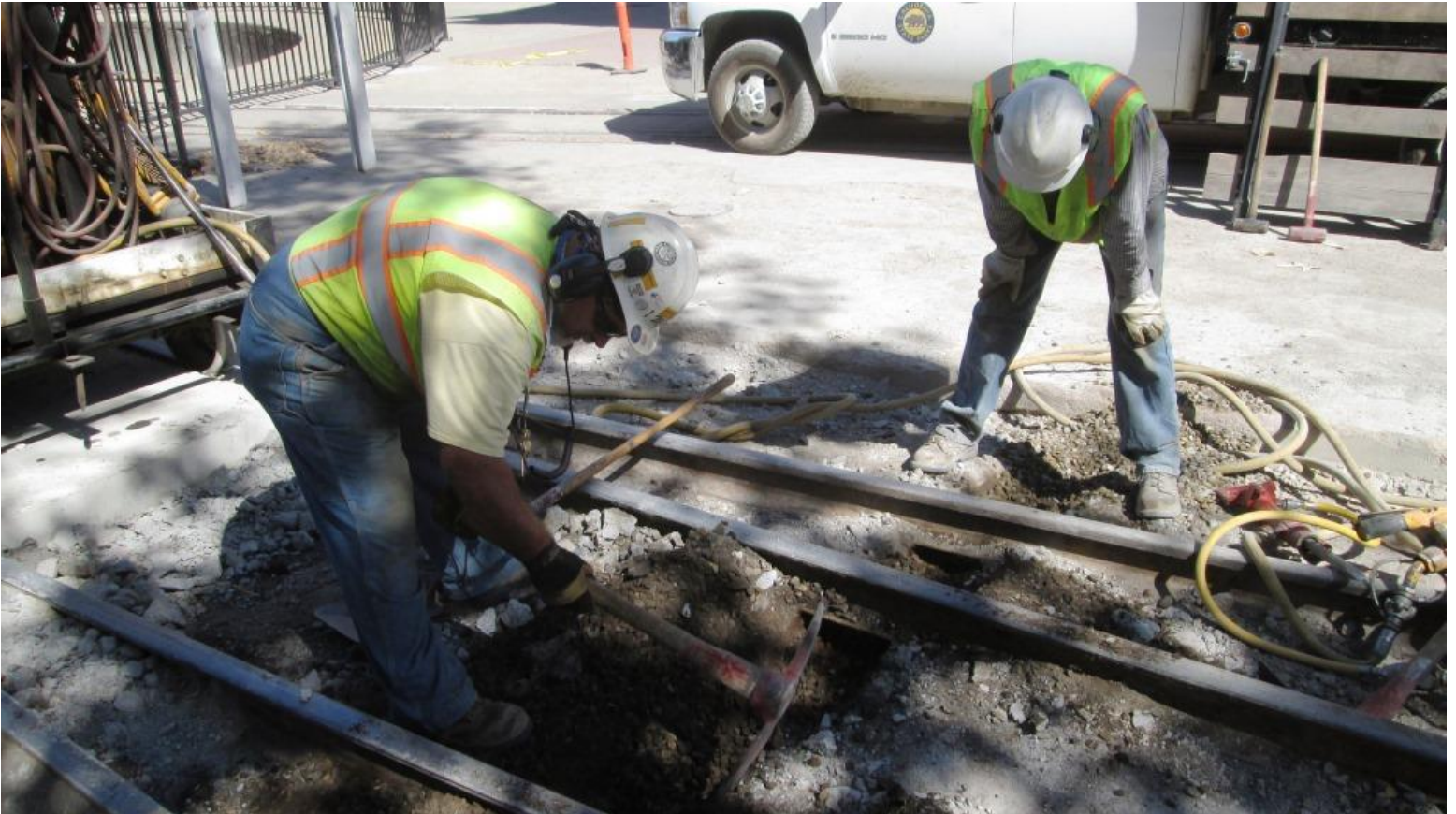
Mike F. and Steve clear space under the rails for the gauge-rod to be installed
