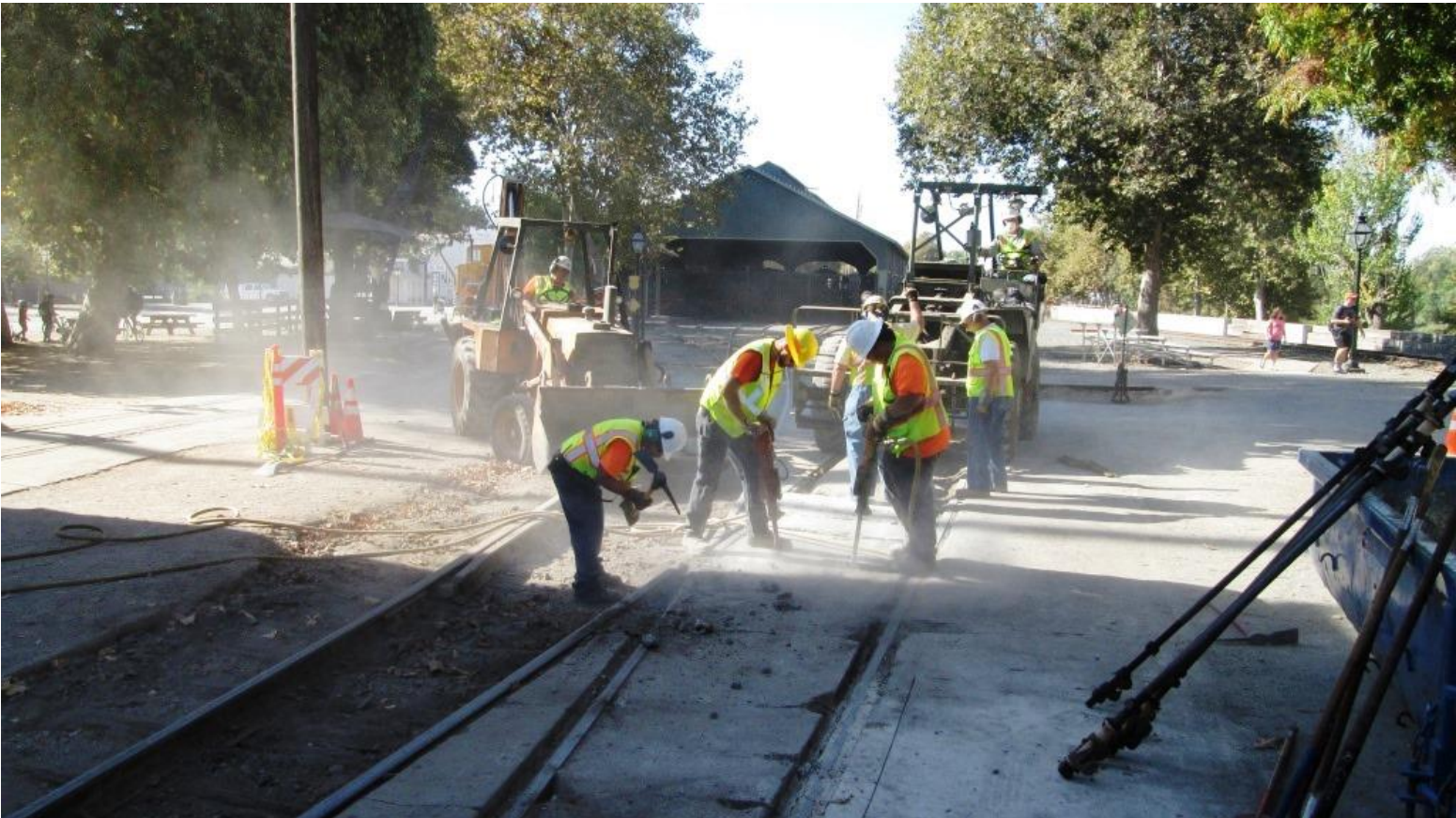
Lots going on here. Harry is on the back-hoe. Steve is on Big Green. Mike and Clem get a concrete slab onto the forks. Chris M. and Anthony jackhammer. Joe breaks out the concrete where the tracks converge with a mattocks
