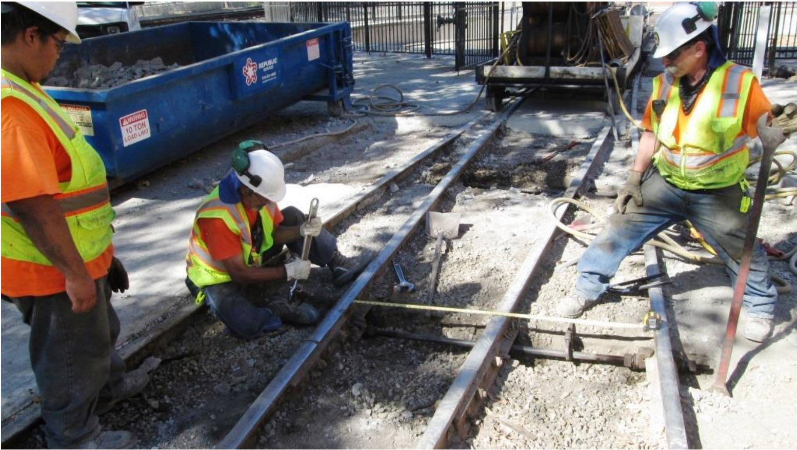
Ed tightens down a clamp on one side of the gauge-rod as Joe stands by to tighten the other
