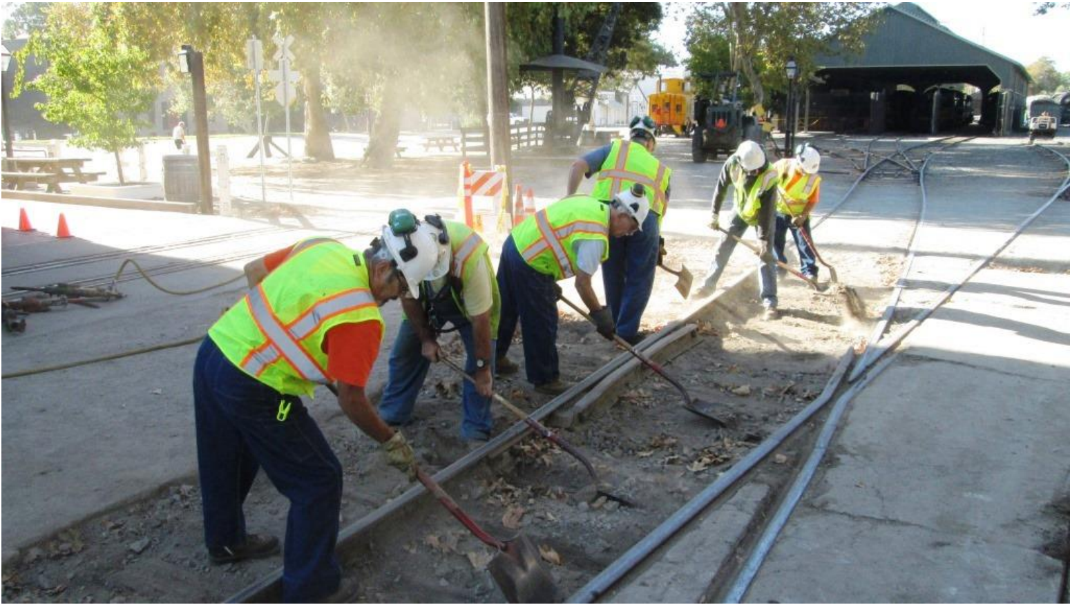
Saturday's work-out commenced with uncovering ties in the area opened up last week
