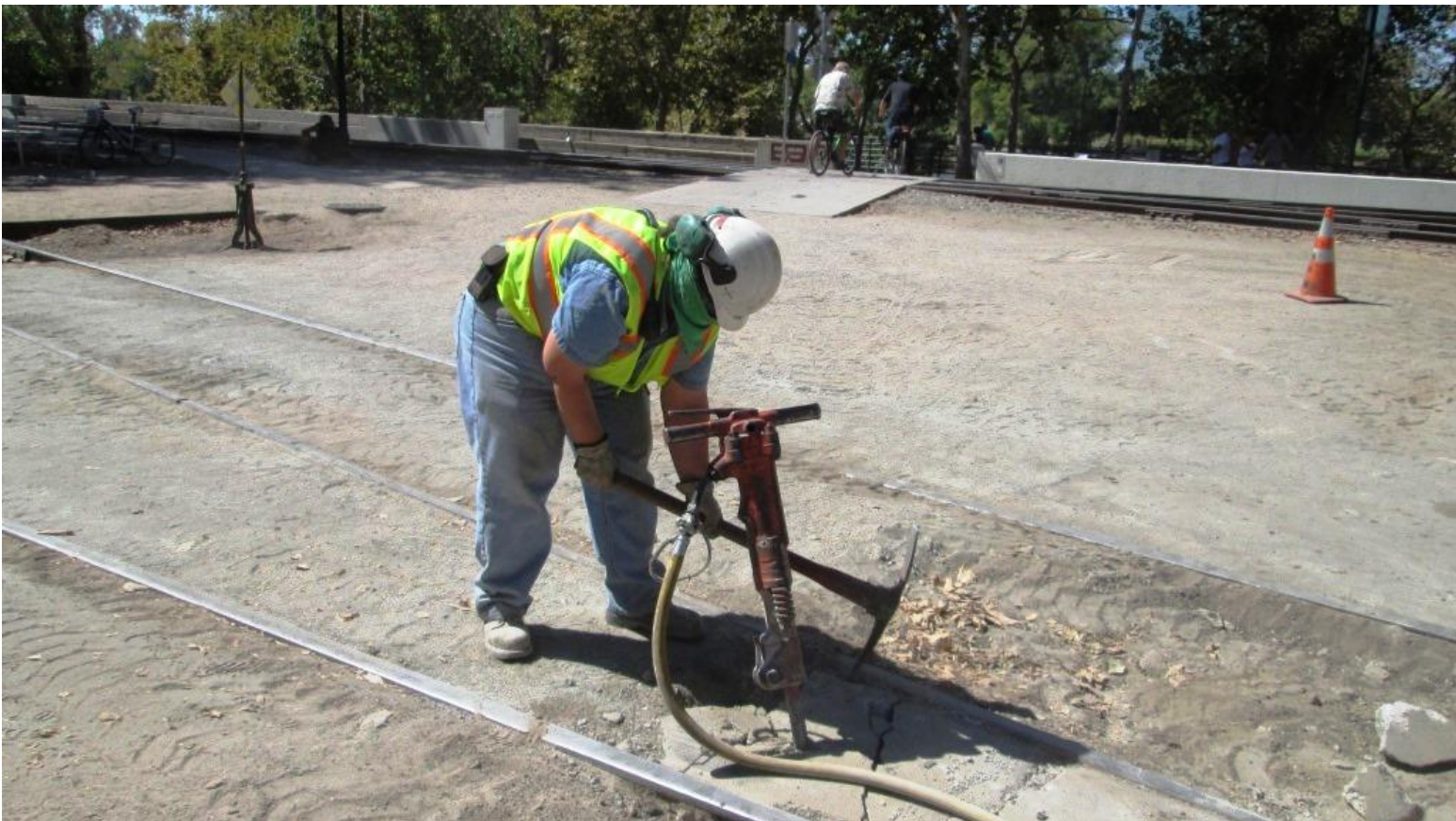
Heather takes on a stuck jackhammer the old fashion way: dig it out by hand...
