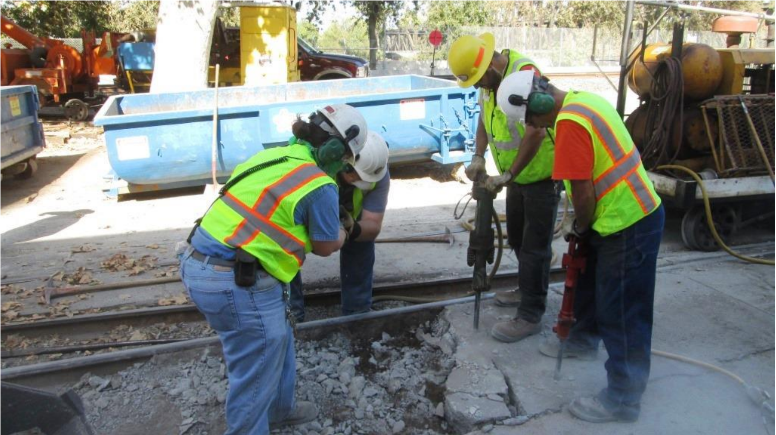
Heather and Chris C. remove concrete debris while Chris M. and Ed continue blasting at it with jackhammers
