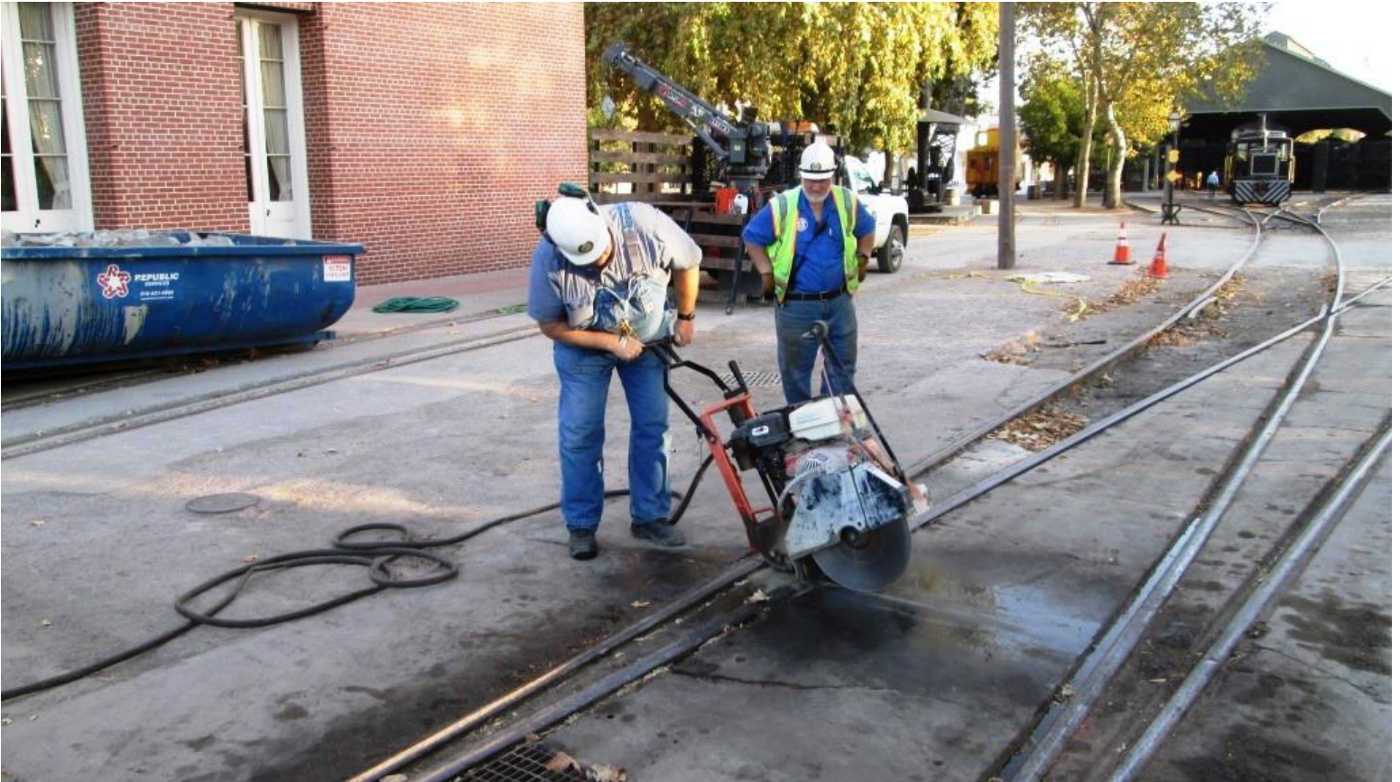
Chris C. and Frank deploy the concrete saw
