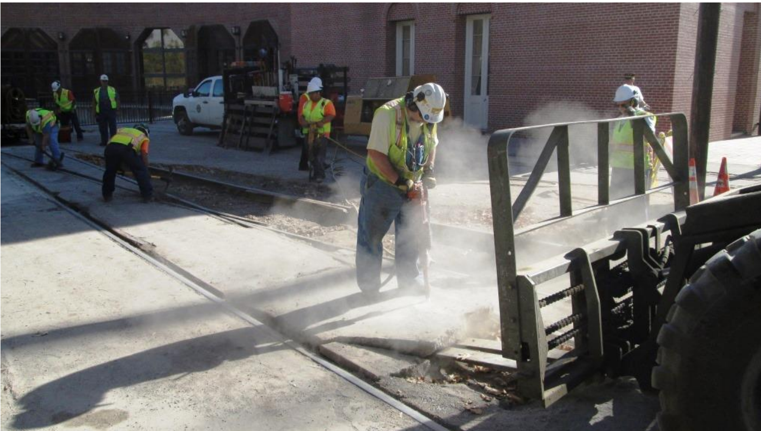
Mike F. uses the jackhammer to chisel off a slab for Steve on Big Green to haul away
