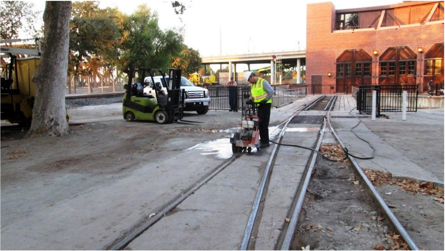
Jose slices concrete along the west rail
