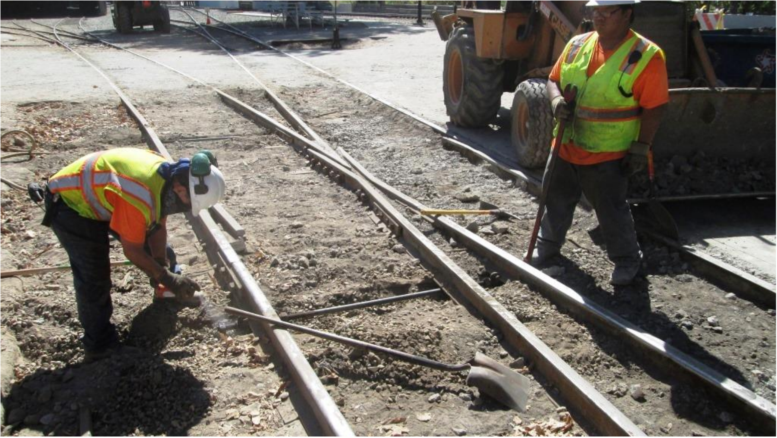
Joe sprays some Kroil on a frozen nut of the gauge-rod
