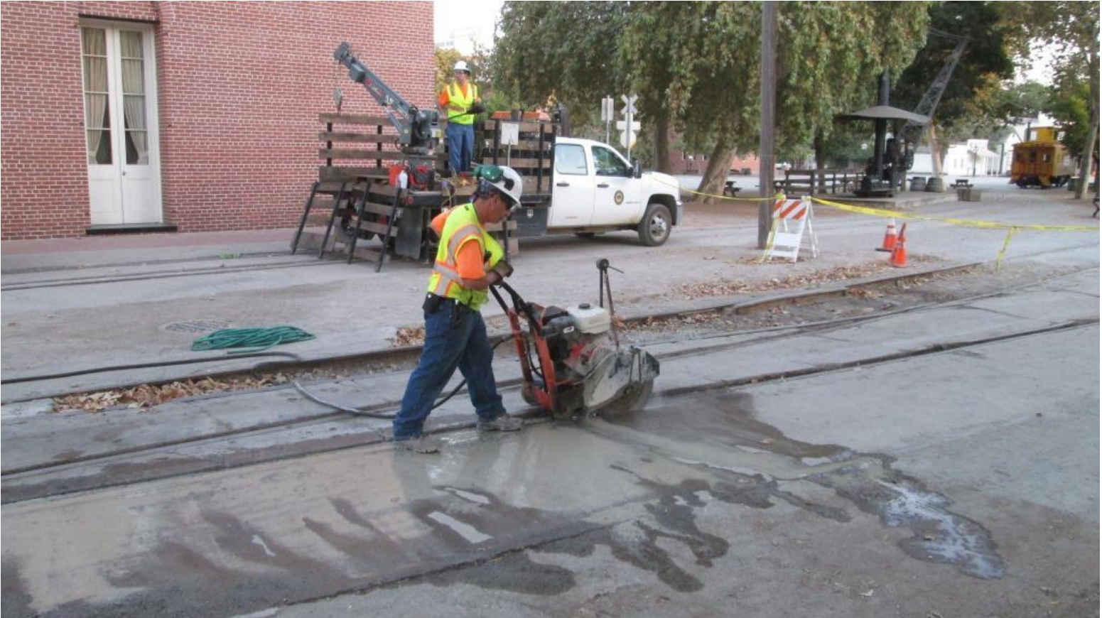
Joe's next on the concrete saw
