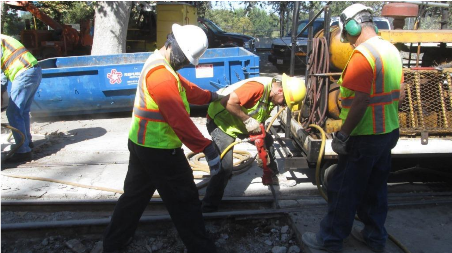
Jose gives Chris M. a helping hand to keep from slipping while chiseling out the cement at the track convergence
