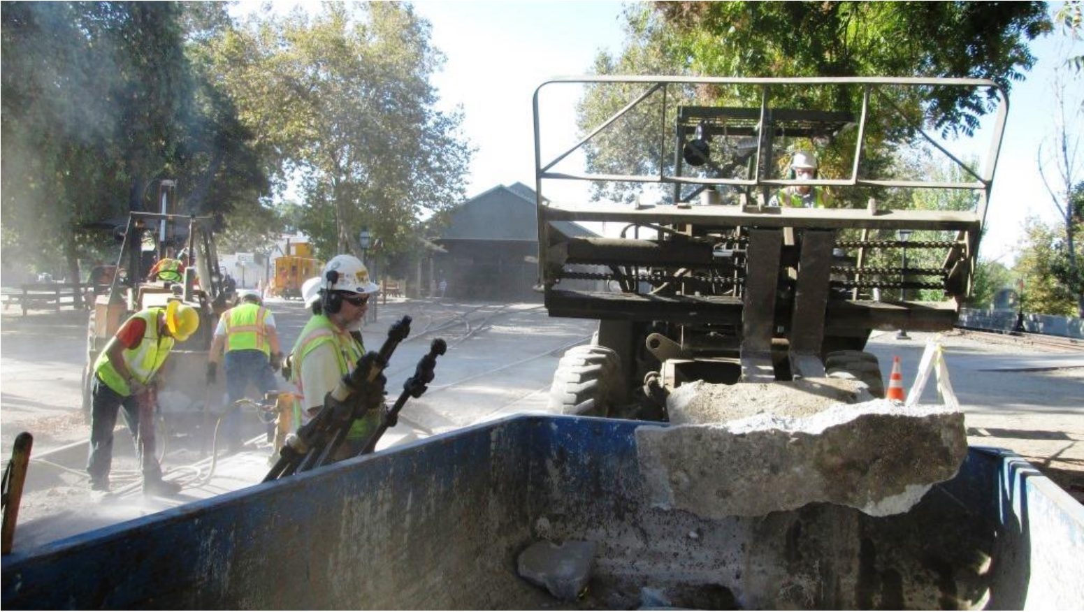
Mike F. guides Steve on the Big Green Machine over to the dumpster to dump large slabs of concrete
