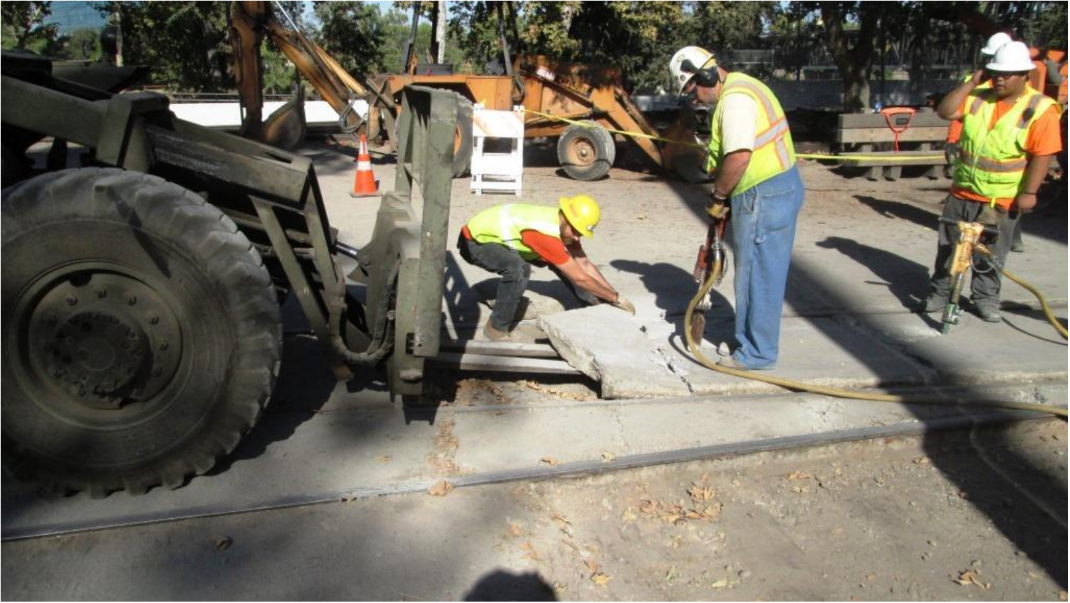
After Mike F. cut through the concrete, Chris M. pulls it onto the forks of Big Green
