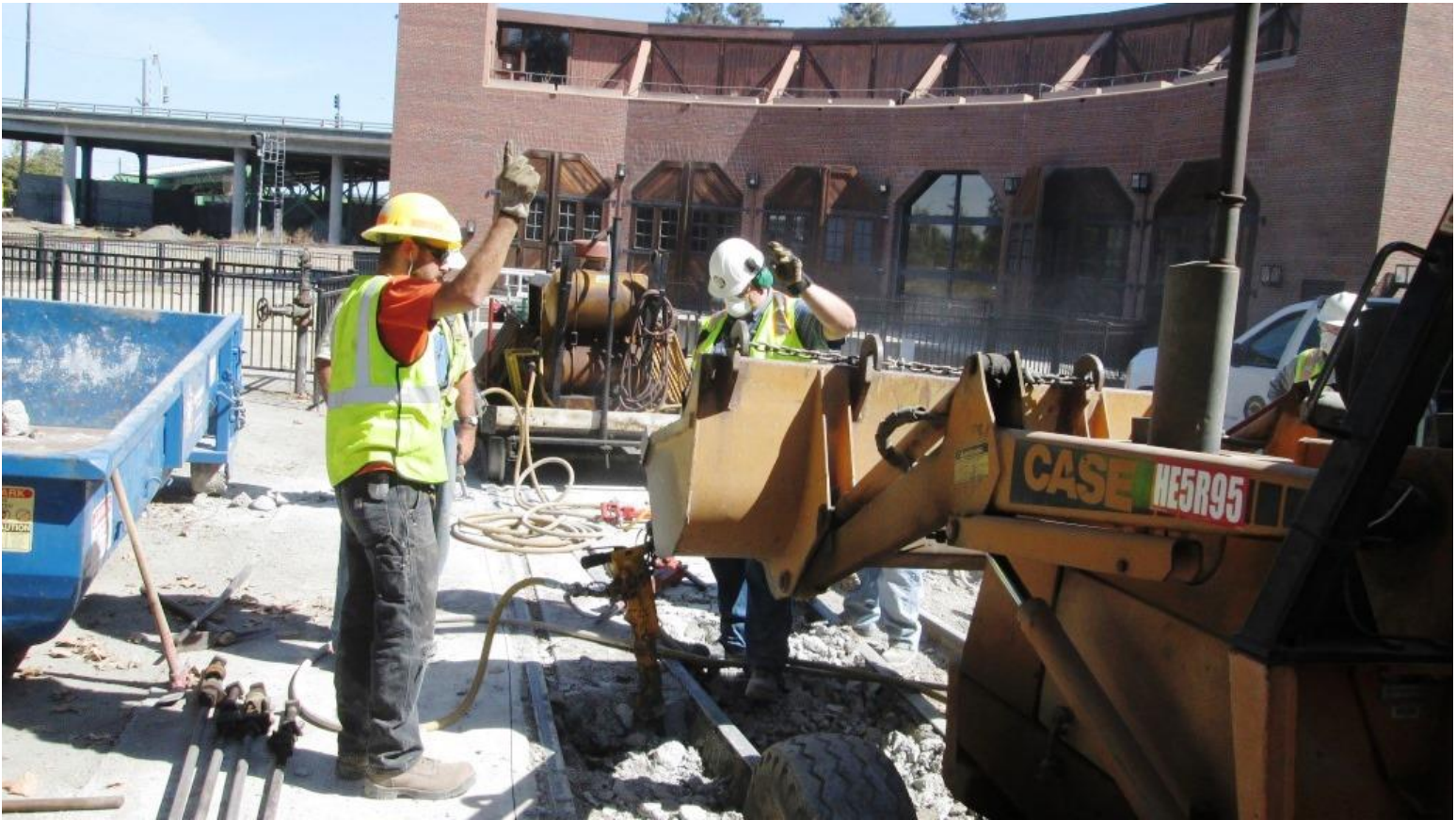
"It's stuck!" Chris M. and Chris C. chain a stuck jackhammer to the back-hoe to pull it out of the ground
