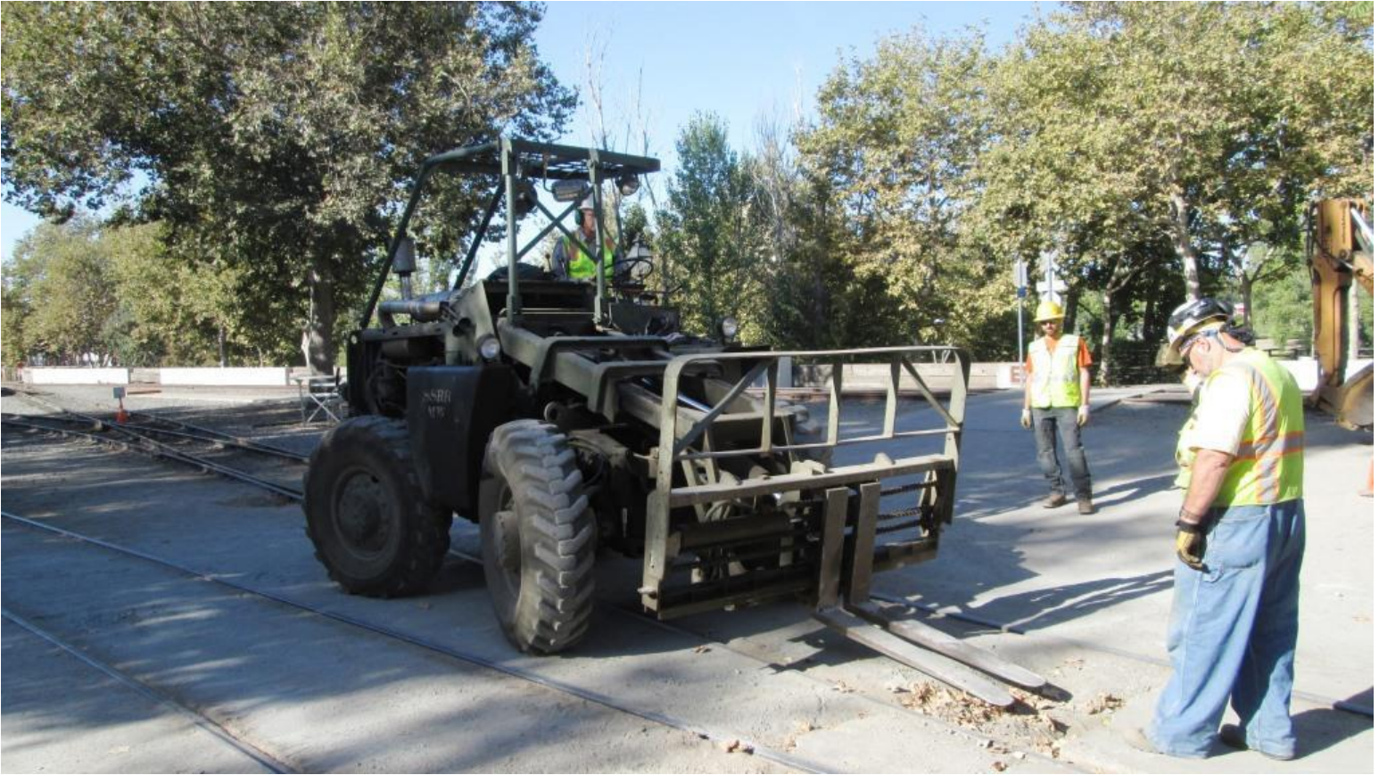
Mike F. guides Steve on Big Green as he gets the forks under the concrete slab
