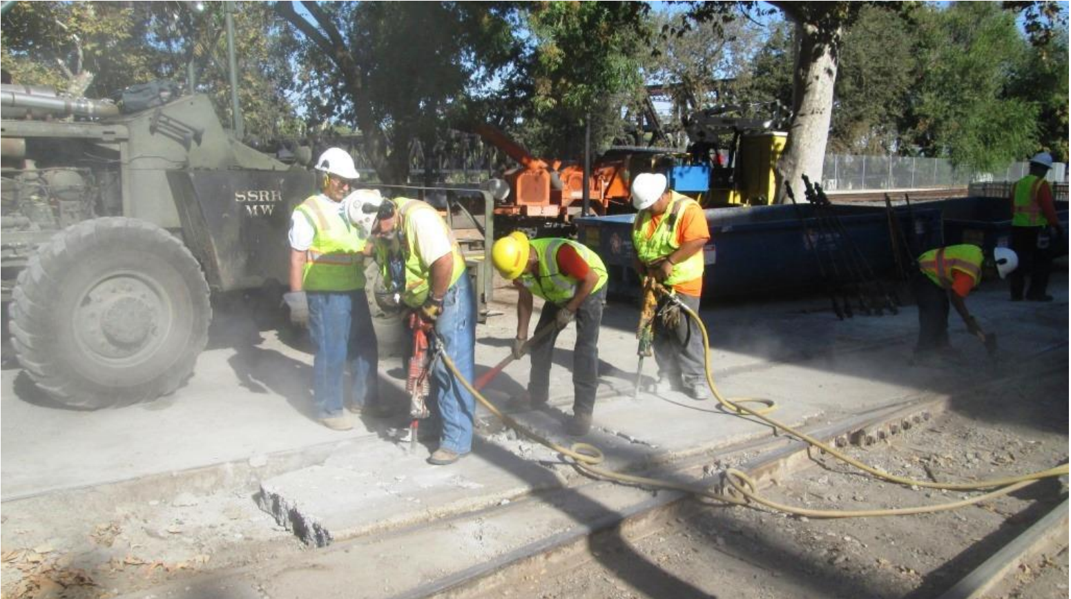
Clem waits to grab some debris while Mike F. and Anthony use jackhammers and Chris M. chips away at the concrete with a mattocks
