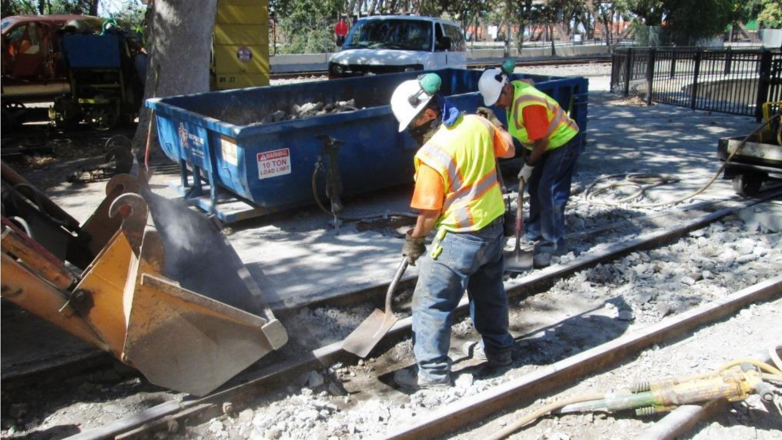
Joe and Ed clean out debris from between the rails
