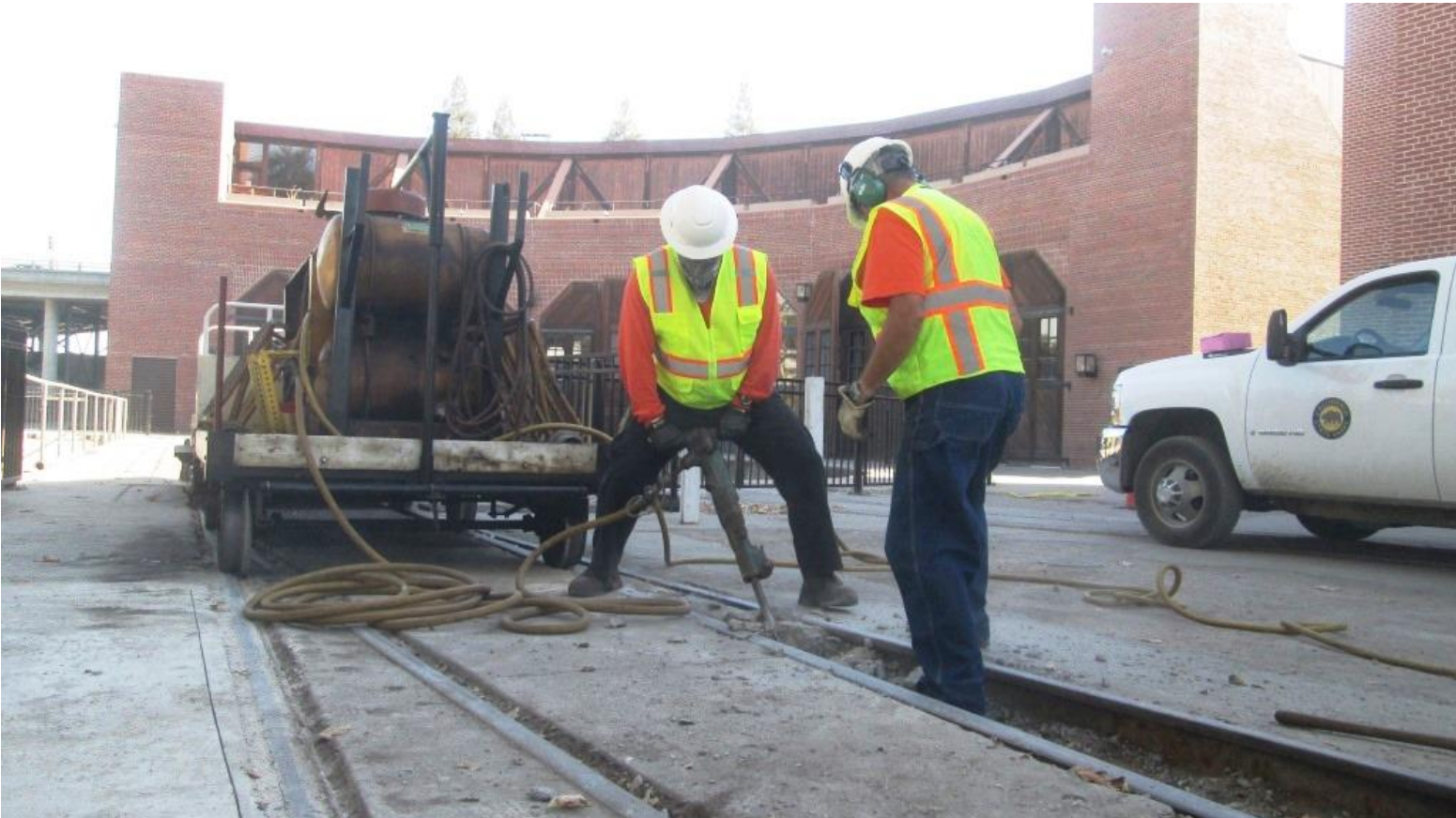
Jose and Ed remove concrete from the track convergence
